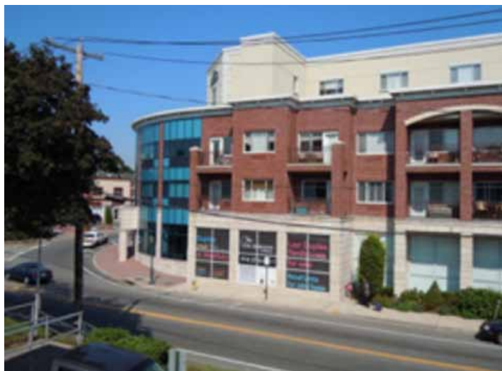
The Horizon mixed-use project across from the LIRR Westbury station
